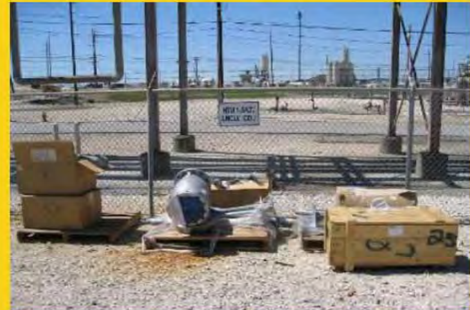
External yards turned to marshalling zones with signs designating areas
